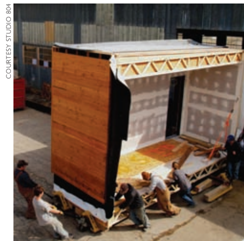
■ The prefab modules hauled out of the warehouse in Lawrence (above) were hoisted onto the Greensburg foundation by crane and then scooted into place by Rockhill and his students (opposite page).
