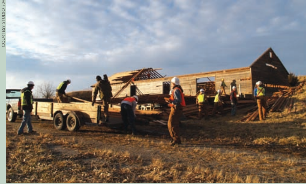
■ Studio 804 scavenged Douglas Fir boards from an abandoned Sunflower Ammunition magazine in early January to form the exterior siding of the 5.4.7 Arts Center.
