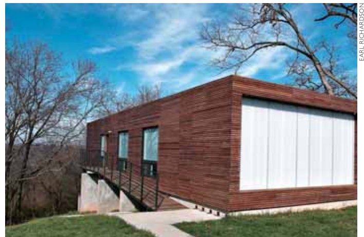
■ Bold design and sustainable building materials like Brazilian hardwood siding won Studio 804 the 2004 Home of the Year award from Architecture Magazine.
