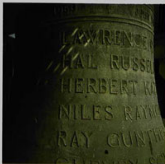
Nearly 50 years ago, the Taylor Foundry in Luttboro, England, cast the carillon's 53 bells from an alloy of pure copper and tin, inscribing them with the names of the 276 KU faculty and students who died in World War II.
