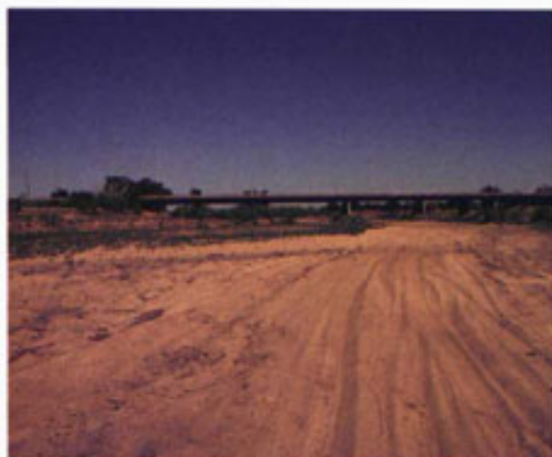
The dry Arkansas River bed, shot in August 1994, with a view of the bridge south of Garden City.
