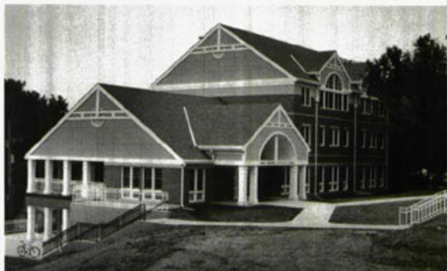
COMFORTS OF HOME: Amini Scholarship Hall brightens the 1300 block of Louisiana Street.
